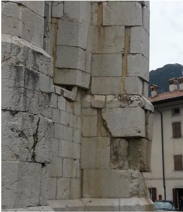
Figure 10. The Duomo di Sant' Andrea Apostolo (Venezia) in Udinese Italy, originally constructed 1261, but substantially from the early 14th century. It was severely damaged by earthquake in 1976. It was reconstructed over 20 years with the active engagement of the local community. The decision was taken to retain evidence of the distortions caused by the earthquake in the reconstructed church, as a reminder of the event and its aftermath, and as a symbol of regeneration within the region. Photo courtesy of Luisa DeMarco.
