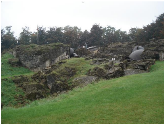
Figure 2a. Fort at Loncin near Liège, Belgium. General view showing the shattered remains of the protective steel domes. Photo courtesy of Stefano F. Musso.
