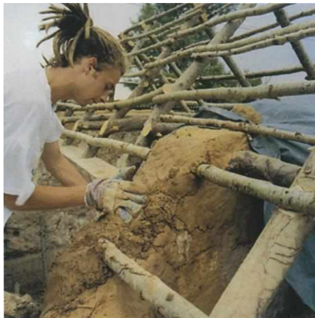
Repairing a mud wall, Poulwitch, Mayglass, Co. Wexford (UCD)
