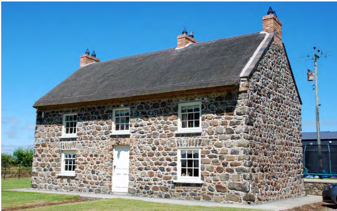
Coursed basalt walls, and thatch, Scroggy Road, Crumlin, Co Antrim (DfC HED)
