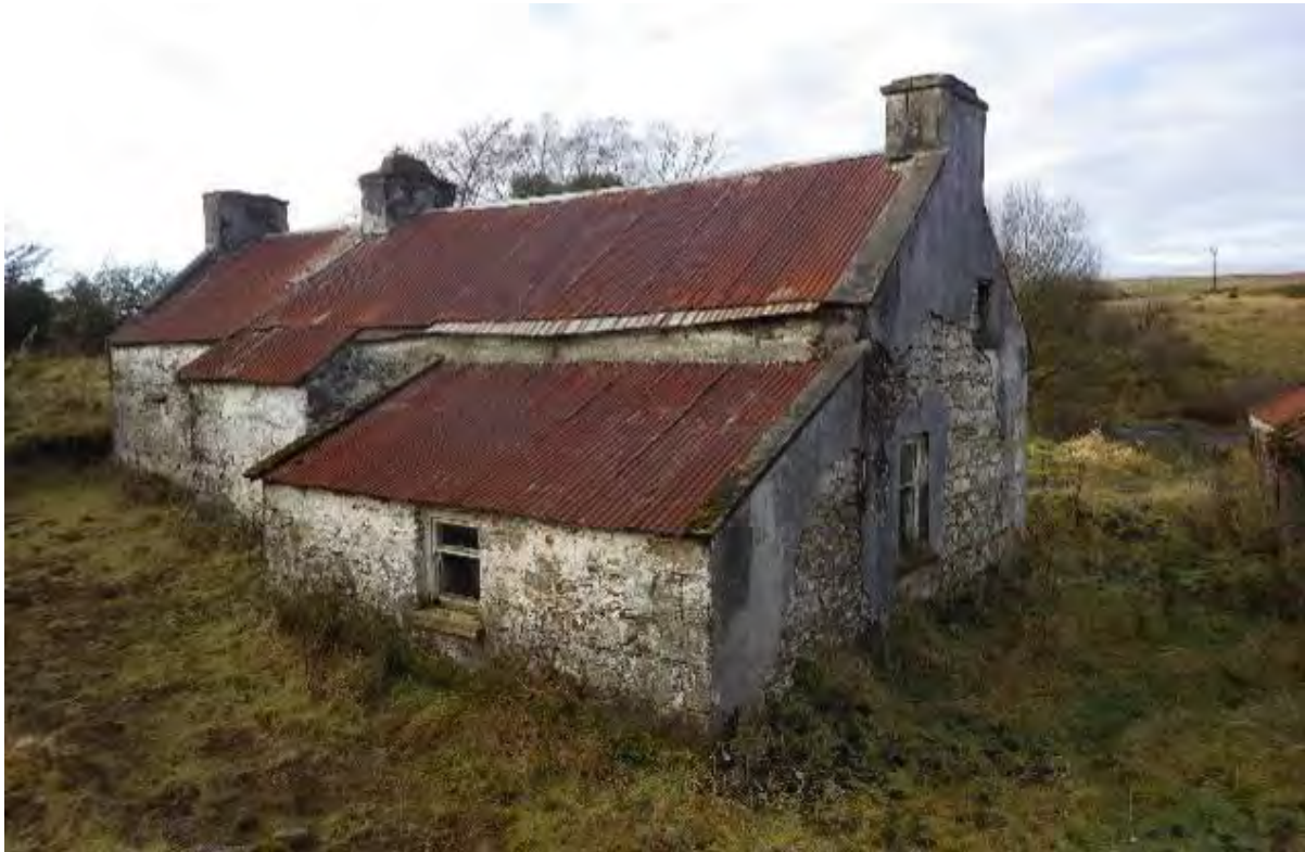
Corrugated iron-roofed house, Scraghy Road, Castleterg, Co. Tyrone with bed outshot projection, typical of the region, at left (DfC HED)
