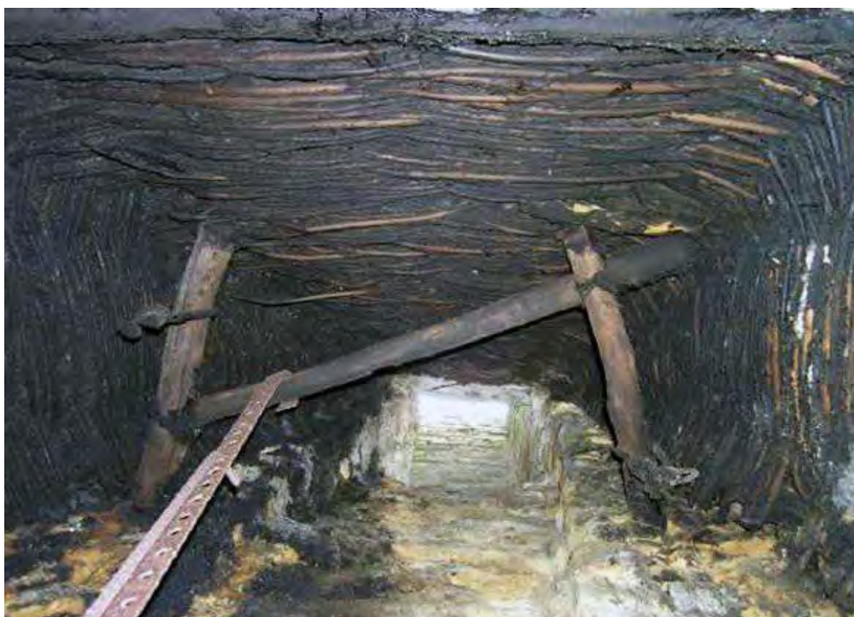
Wickerwork chimney, Slievecorragh, Co. Wicklow (Christiaan Corlett)
