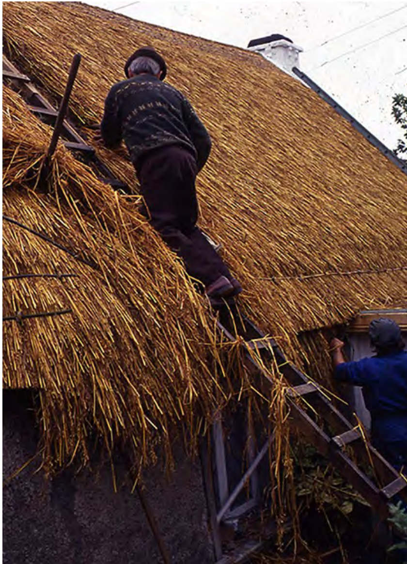
Rethatching in progress, Commons West, Swords, Co. Dublin (Barry O'Reilly)
