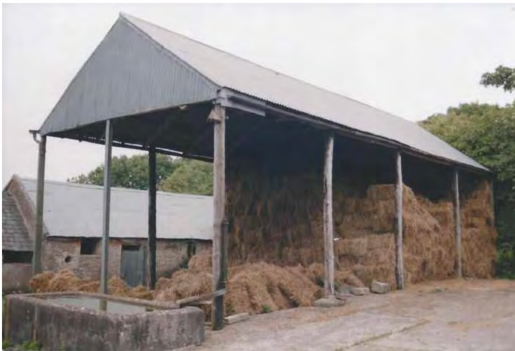
Hay barn of vernacular character, with timber pole supports and pitched roof, Maddyboy, Barringtonsbridge, Co. Limerick (Barry O'Reilly)
