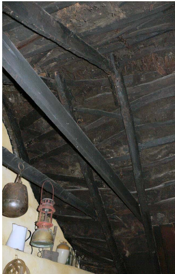
Typical A-frame roof structure at Lisnacon, Kanturk, Co. Cork (Barry O'Reilly)
