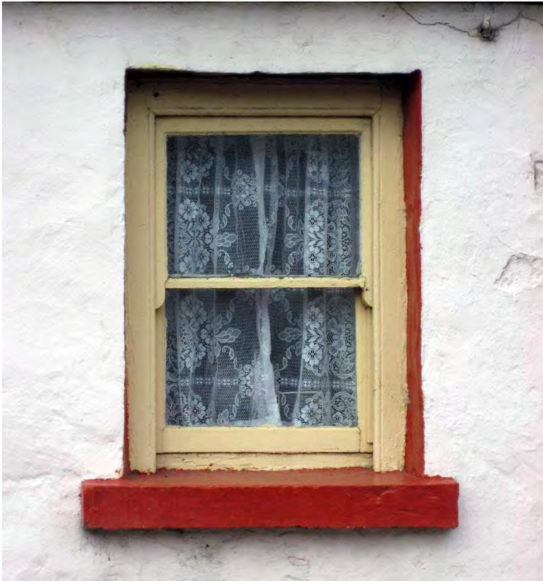
Typical sliding sash window at Tober Hill Street, Westport, Co. Mayo (NI)
