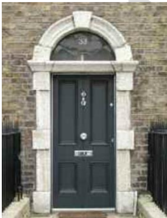
Figure 50 Aluminium draught strips can be seen to all sides of this door. The metal part of these strips, unfortunately visible, can be painted but it is important that the flexible sealant strip is not.
