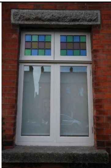
Figure 73 Timber framed window (copyright lambstongue.ie).
