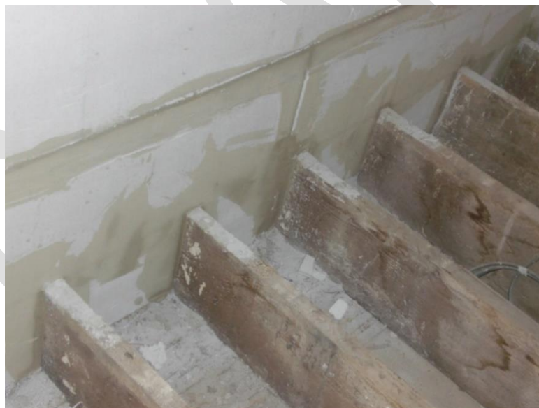
Figure 55 Calcium silicate boards applied to walls and carefully fitted around and between floor joists to ensure continuity of insulation.
