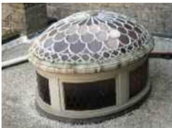
Figure 40 Historic skylights and lanterns, such as this fine example, should be well-maintained but are rarely suitable for thermal upgrading.
