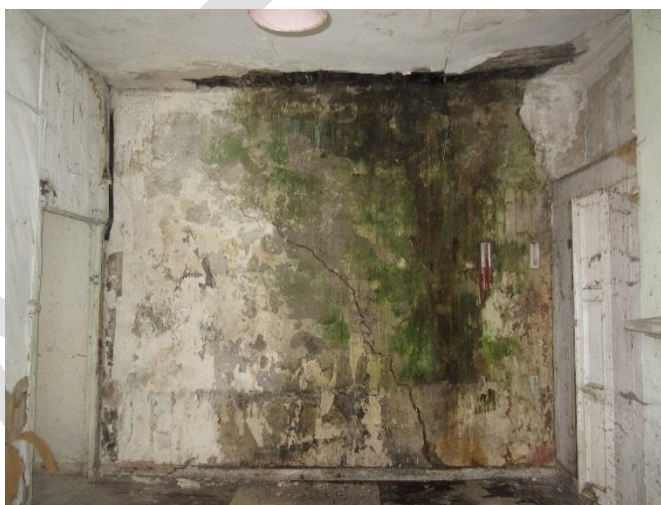
Figure 17 Extreme case of mould growth.
