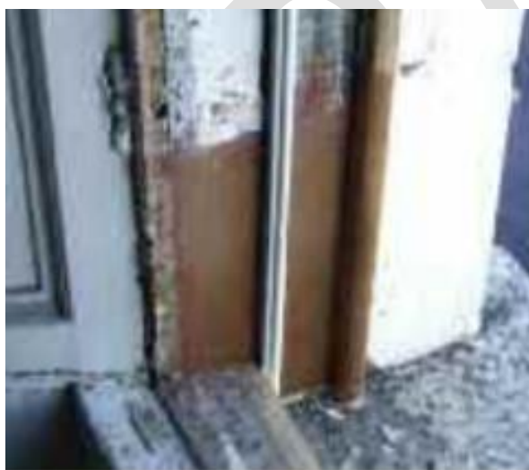
Figure 47 A repaired window frame with a replaced style and new parting bead. The timber sash frames have been temporarily removed.
