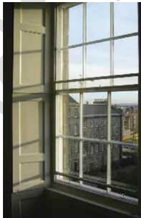
Figure 51 Carefully designed bespoke secondary glazing installed as part of Changeworks' Energy Heritage project.
