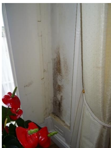
Figure 16 Mould growing behind shutters.
