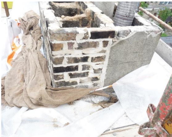
Figure 38 Repointing of bricks with lime-based pointing after removal of cement render.
