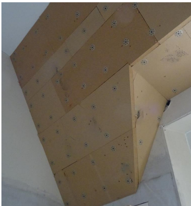
Figure 35 Woodfibre insulation board fixed to directly to the internal face of rafters of the coombe. This would only normally be done if a woodfibre sarking boards cannot be installed to the external face of the rafters.
