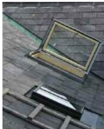
Figure 41 This modern double-glazed skylight allows access to a concealed valley gutter for maintenance inspections and cannot be seen from ground level. It also lets additional natural light into the attic space below.
