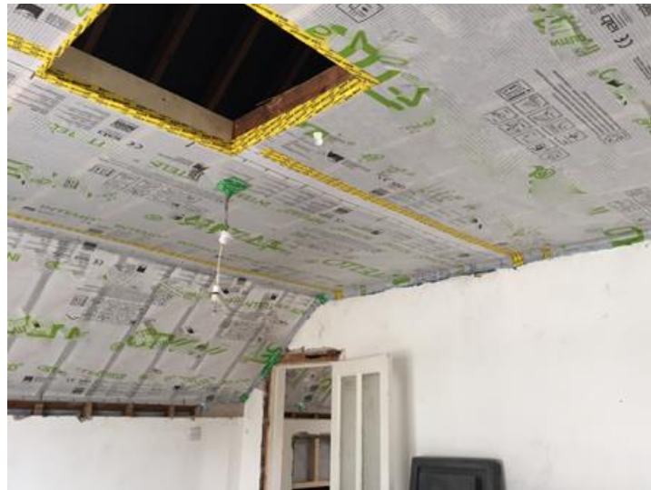
Figure 32 Vapour control membrane fitted to the warm side of the insulation to reduce vapour transfer from the room below.
