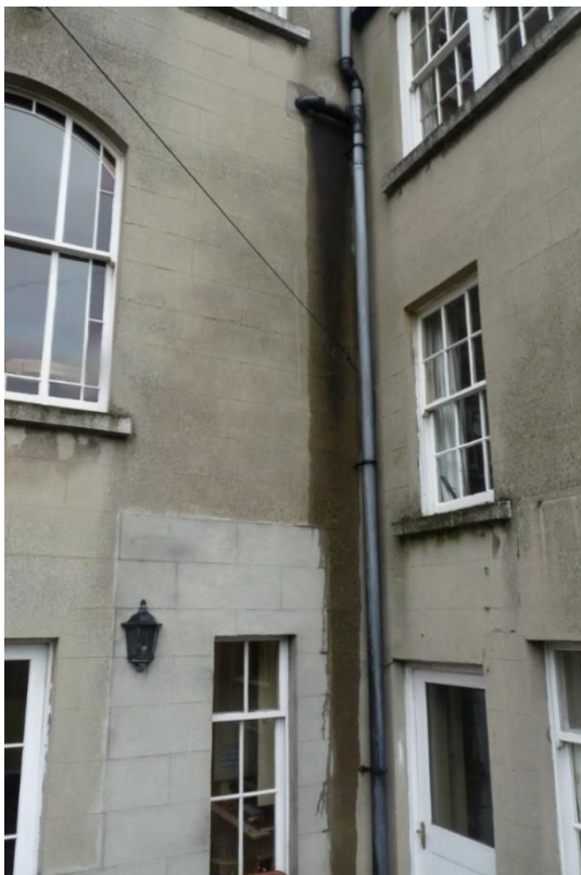
Figure 27 Example of cement render applied to a traditional building. Water from a leaking drainpipe can penetrate the cement render and increase moisture build up in the wall. This can lead to rot in any timber elements in contact with the wet masonry.
