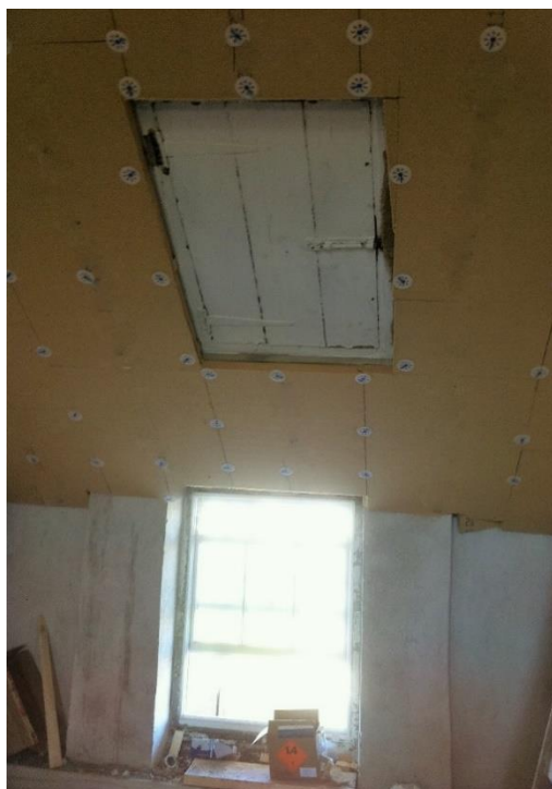
Figure 34 Woodfibre insulation boards fixed over roof insulation and cut around attic hatch. The attic hatch must also be insulated as far as possible to minimise thermal gaps.
