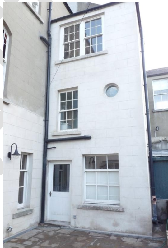
Figure 28 Same building with the drainpipe leak fixed and the cement render replaced with a traditional moisture permeable lime render.
