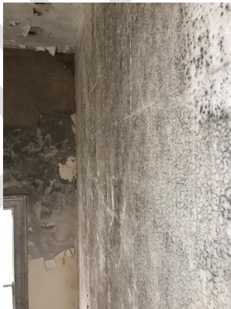
Figure 10 An example of a consequence of poor moisture movement through building fabric. Materials which trap moisture can increase the risk of mould growth.
