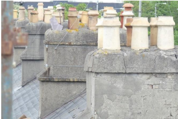
Figure 36 Traditional chimneys, some with added cement render.
