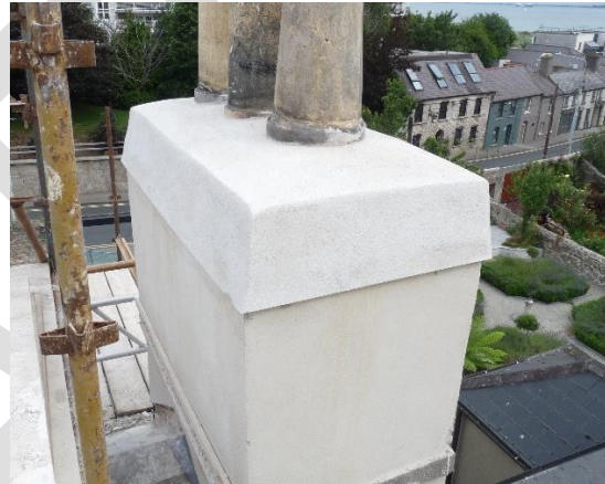
Figure 39 Almost completed chimney, with existing cement render replaced with lime render.
