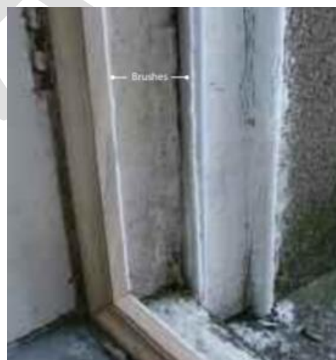
Figure 48 Draught-proofed window frame: brushes are visible on the staff and parting beads, both of which have had to be replaced in order to draught proof. For the brushes to work properly it is important that they are not painted over.
