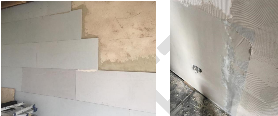
Figure 53 Calcium silicate insulation boards installed internally (left) over a mesh layer of skim finish (right).
