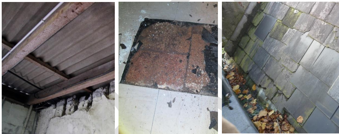
Figure 19 Examples of where asbestos can be found – panels of corrugated roof sheeting, floor tiles and roof tiles.
