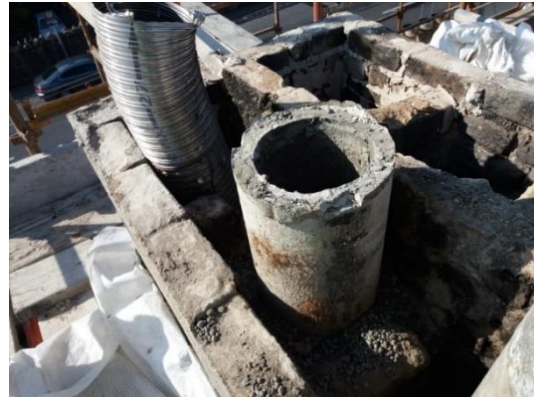
Figure 37 Temporary removal of chimney to rebuild bricks.
