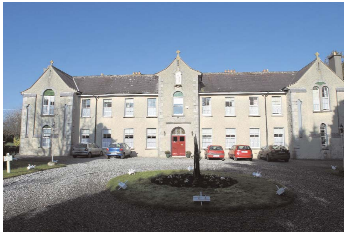
(fig. 174) ST MARY'S CONVENT St Mary's Road Edenderry (1916)
