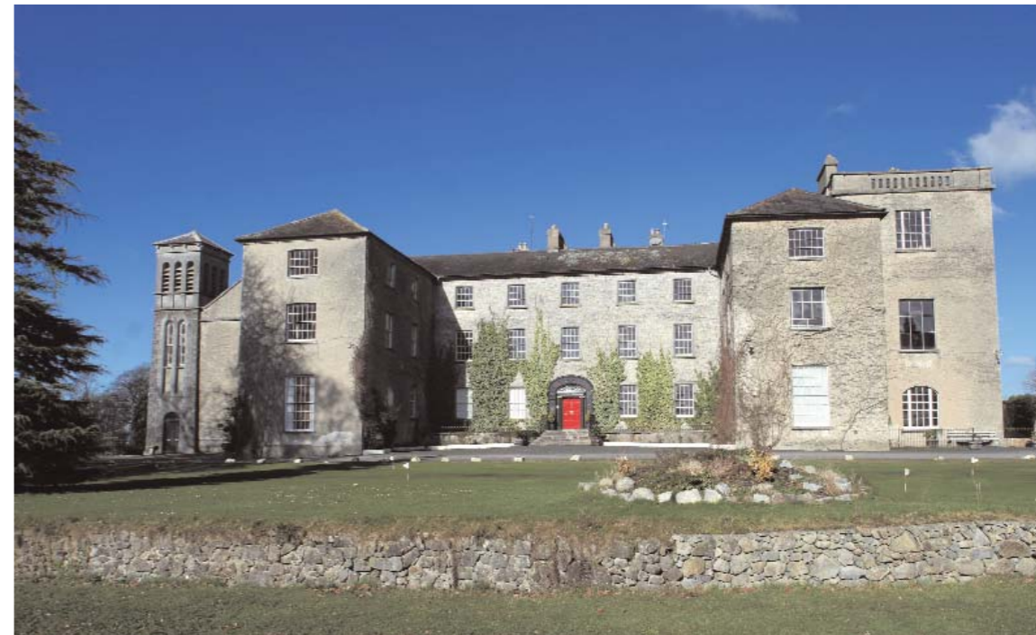
(fig. 56) ST STANISLAUS CATHOLIC COLLEGE Tullybeg (1815-18)
