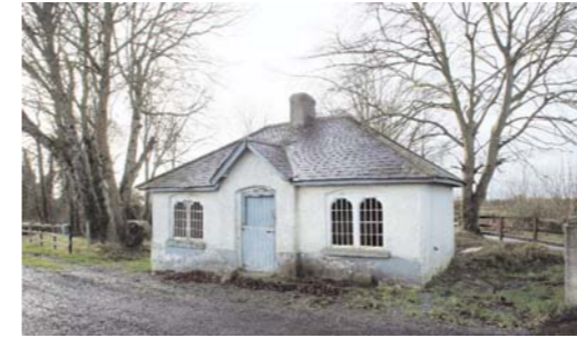
(fig. 99) KILCLONCORKRY HOUSE (c. 1820)
