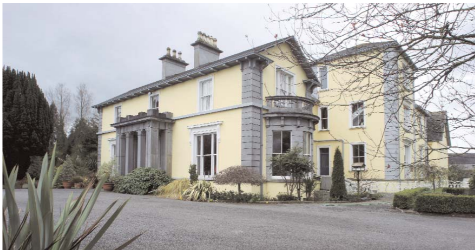
(fig. 130) INCHMORE HOUSE Kilcoursey Clara (c. 1860) Designed for the Goodbody family by the architect John Skipton Mulvany. Several features such as the heavy stone portico, curved, rusticated bay with balcony and roof with wide eaves, are typical of this architect's style.
