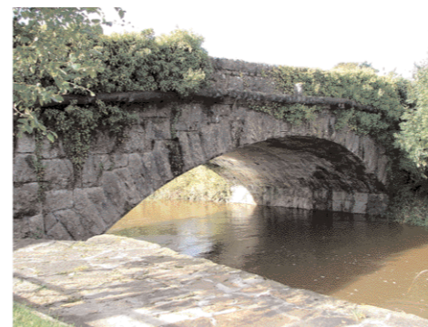
BALLYCUMBER BRIDGE Ballycumber (c. 1850)
