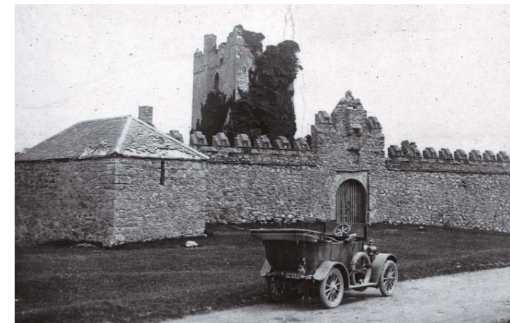
(fig. 5) CLONONY TOWER- HOUSE Clonony More (c. 1500)
