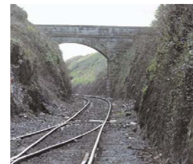
GAOL BRIDGE Tullamore (c. 1859)
