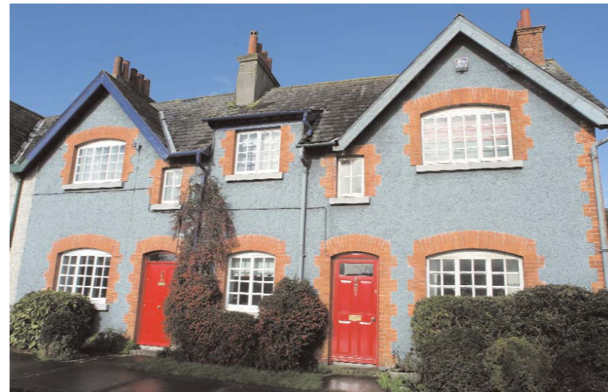
( fig. 171 ) 20-21 CONVENT VIEW TERRACE Tullamore (c. 1900)
