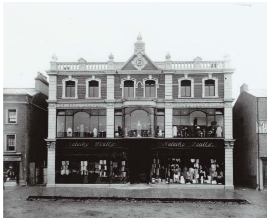
(fig. 179) SCALLY'S Columcille Street Tullamore (1911-14)
