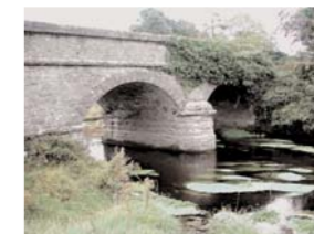
KILCUMBER BRIDGE Kilcumber (c. 1850)
