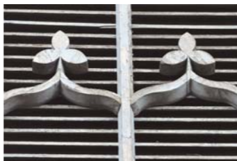
ST BRENDAN'S CHURCH Detail of decoration on the wooden louver.
