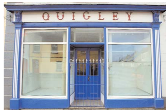
QUIGLEY This symmetrical shopfront has centrally placed half-glazed doors and retains many of its original features, including the cast-iron gate.
