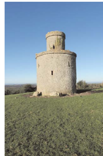
(fig. 78) SADLIER'S TOWER Killurin (c. 1820)
