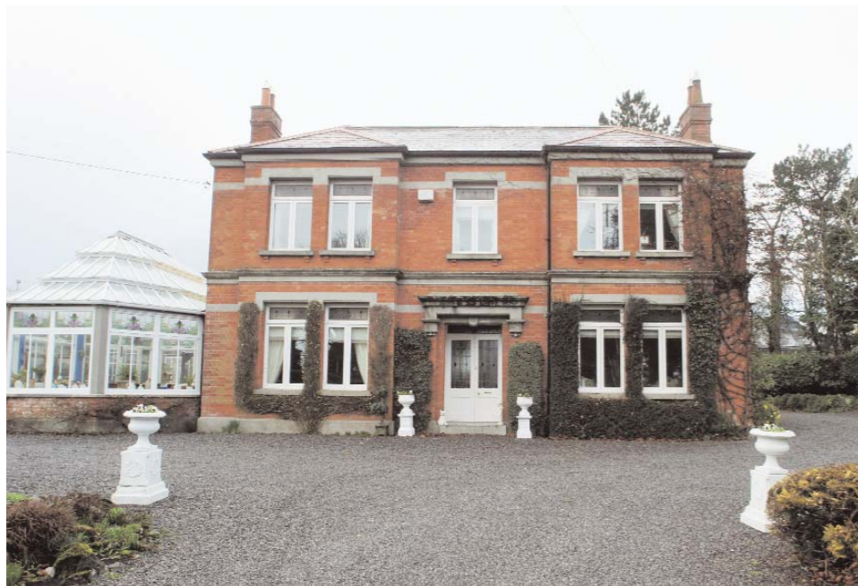
(fig. 172) KILLEIGH ROAD Tullamore (c. 1900) A substantial red brick suburban house, which has handsome details, is typical of houses that were being built for the professional classes in the early years of the century.
