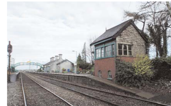
TULLAMORE RAILWAY STATION Tullamore (c. 1855)
