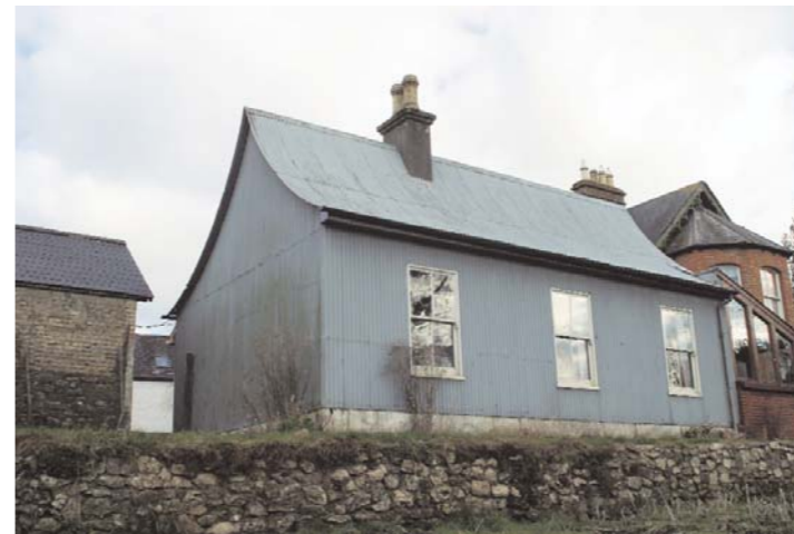
(fig. 139) BEECHMOUNT HOUSE Kilbeggan Road Clara (c. 1880)
