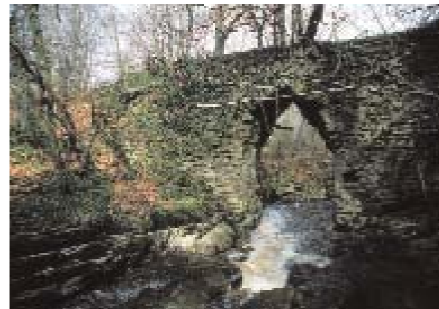
(fig. 3) CASTLEFIELD BRIDGE Cadamstown (c. 1500)
