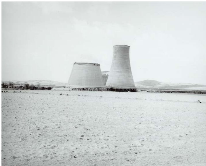
(fig. 181) ESB POWER STATION Rhode (1956-63)
