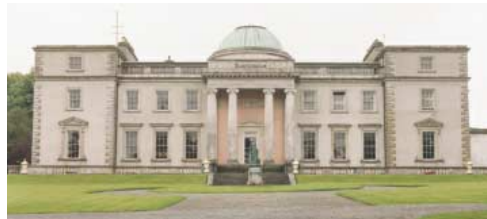
The Garden Front as eventually executed is not unlike the Entrance Front but with a portico without pediment, completed by Lewis Vulliamy c. 1835. The dome was completed, c. 1860.
