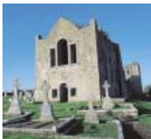
(fig. 8) OUGHAVAL CATHOLIC CHURCH, Stradbally (c. 1500)
