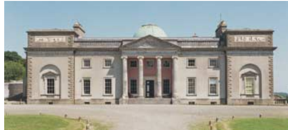
(fig. 19-28) EMO COURT, Emo (begun c. 1790). The Entrance Front, completed c. 1798, is much as Gandon intended although the hipped roofs and drum to dome are well concealed by panelled and balustraded parapets.
