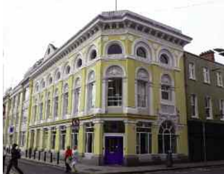
(fig. 96) AXA (formerly Beakey & Co. Warehouse ) Wolfe Tone Street/12-13 Mary Street (1863)
