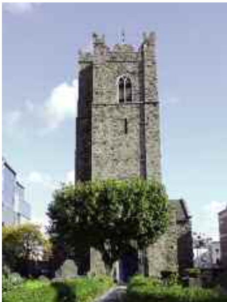
(Fig. 5) ST MICHAN'S CHURCH Church Street (1685)
