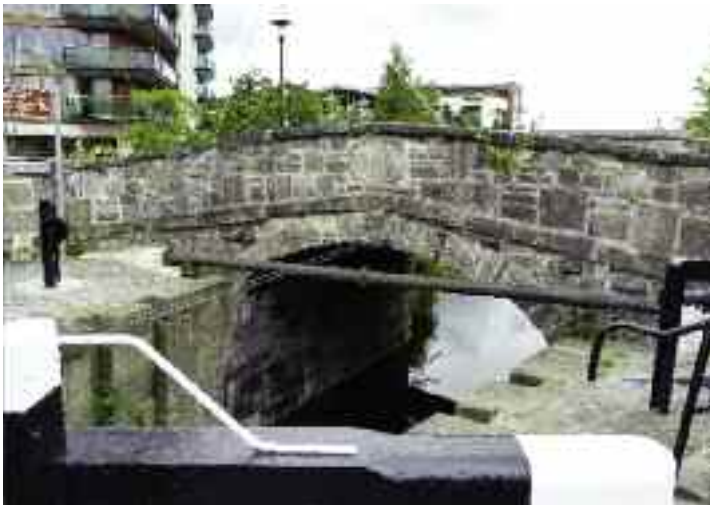
(fig. 36) ASHTOWN BRIDGE (formerly Longford Bridge) (1792)
