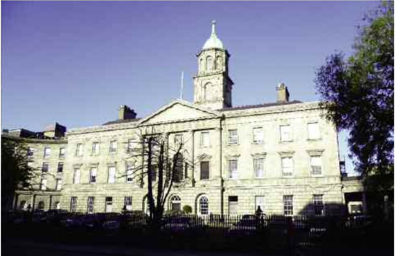
(fig. 21) ROTUNDA HOSPITAL Parnell Square (1751-7)
