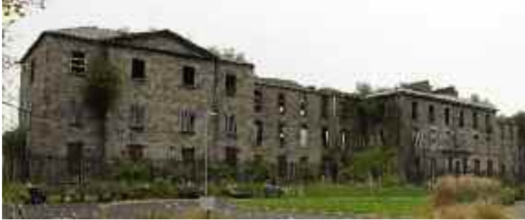
(fig. 57) ST BRENDAN'S HOSPITAL Fitzwilliam Place North/Morningstar Avenue (1810)
