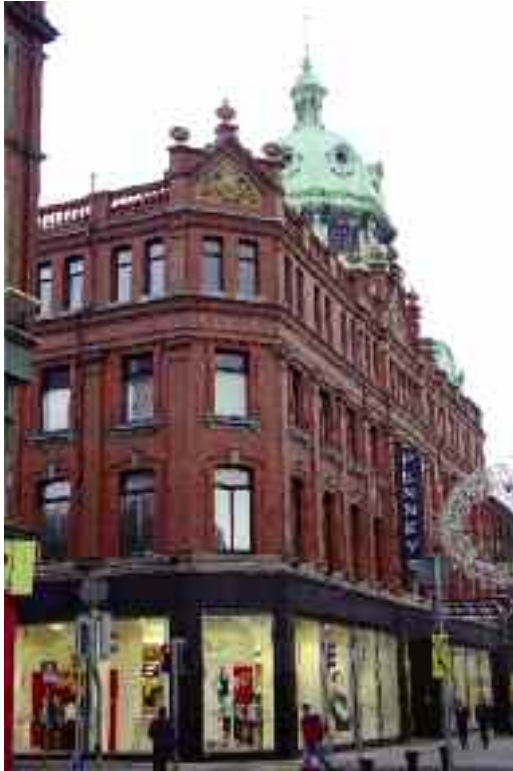
(fig. 97) PENNEYS (formerly Todd Burns & Co.) 45-47 Mary Street (1902-5)
